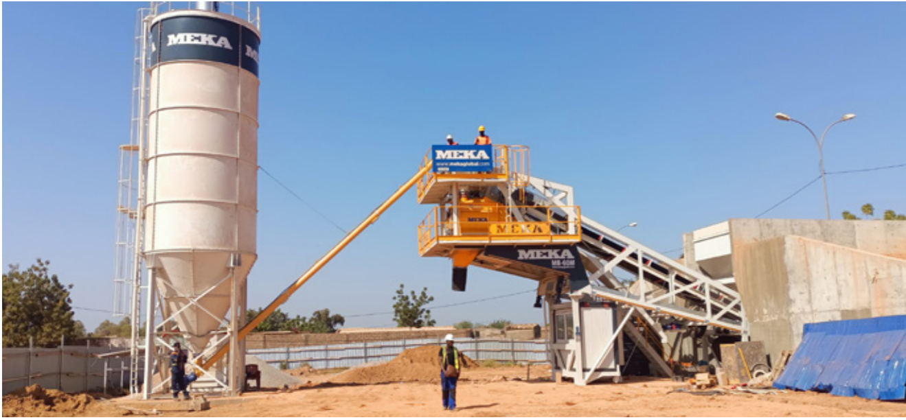
▲ Meka Mobil Beton Santrali Kurulumu-2024 Burkina Faso
